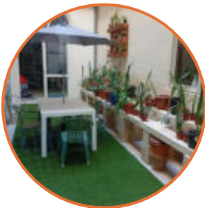
Fra Diegu internal yard refurbishing
